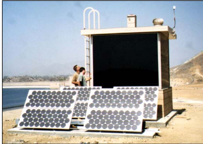
Figure 6. Observing station TS4, on the West Dam
